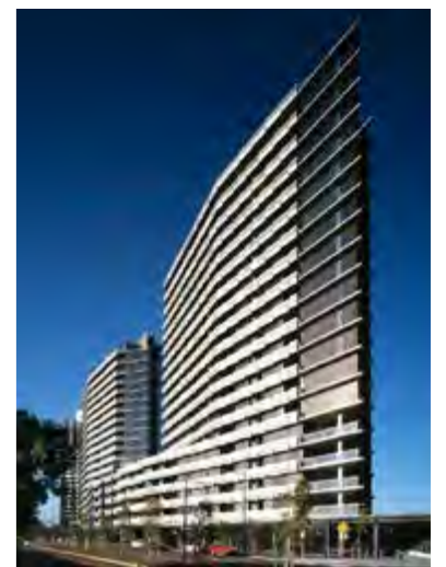
WATERGATE TOWERS Waterview Walk, Docklands 350 apartments and retail
